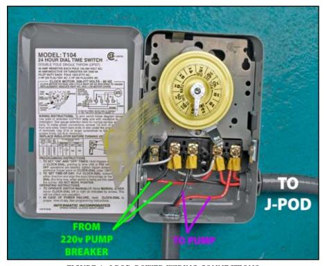
FIGURE 1 J-POD POWER WIRING CONNECTIONS
